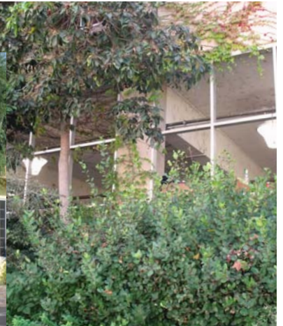
Nationwide Auto Detailing, first floor Sater Parking Structure
